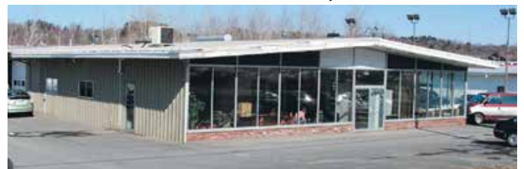
Central Maine Reconditioning Center 23 Airport Road, Waterville
