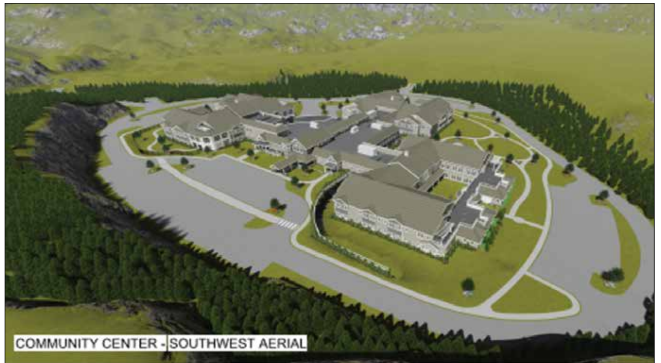
An artist rendering of the aerial view of the new Maine Veterans' Home in Augusta.
